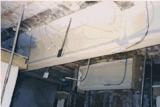
beam before fire test
